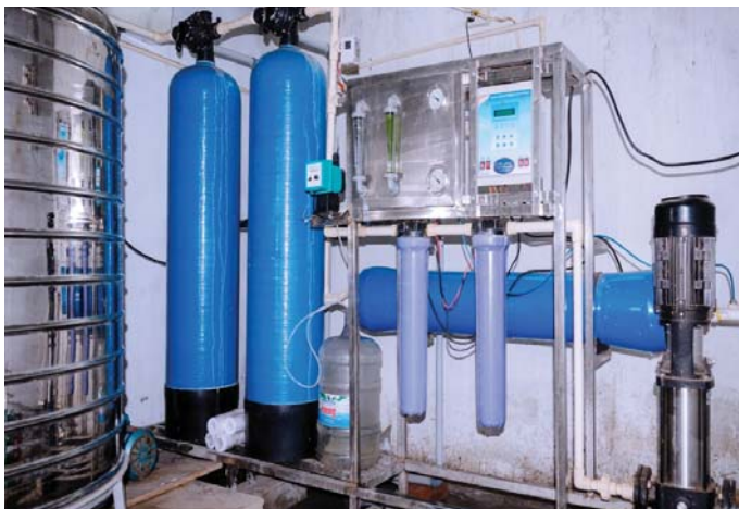
RO WATER PLANT
